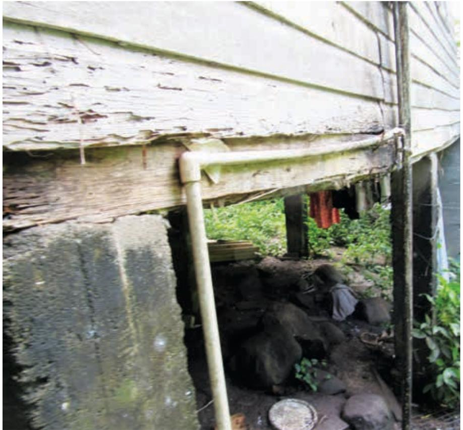
*The wooden beams and cement supports of an old home are deteriorating.*
